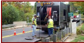
Sewer inspection (above); Utility line maintenance(below)
