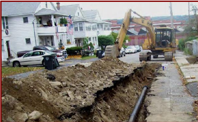
Installation of new water main
