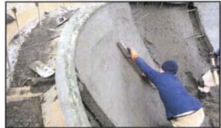
Ecosmart Concrete over crushed recycled concrete sub base
