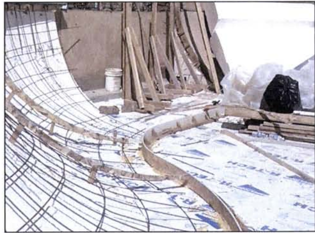
Light-Weight Structural Styrofoam Sub Base Queensborough All-Wheel Park - New Westminster, BC and Seattle Center Skate Plaza - Seattle, WA
