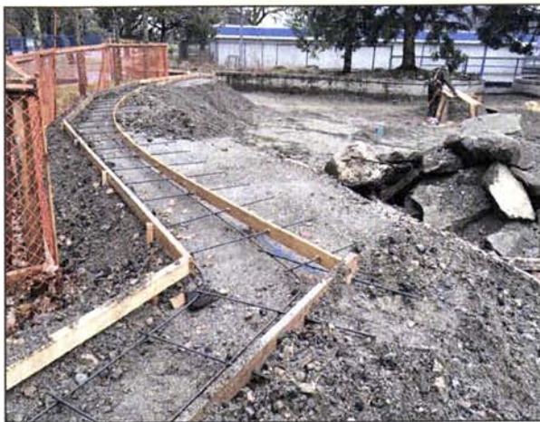
Re-Use of Original Concrete Slab, Sub Base, and Drainage Structures Ambleside Skatepark Replacement - West Vancouver, BC
