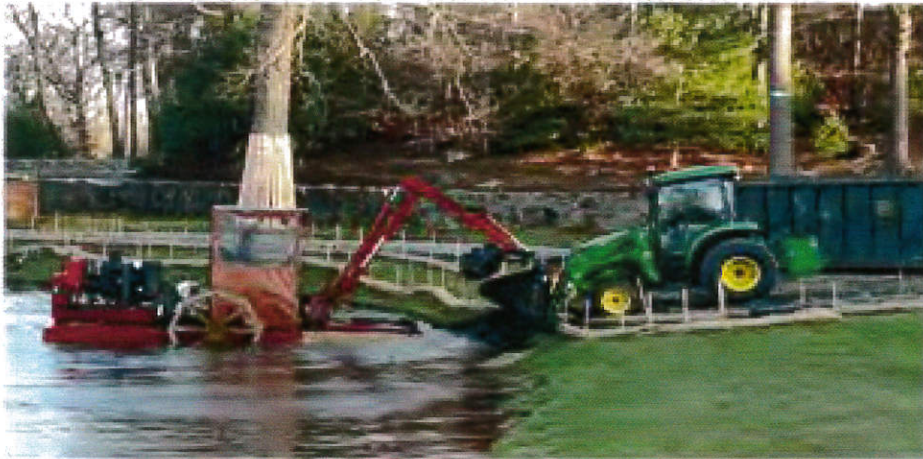
Image 2: Typical hydro rake and front-end loader operation
