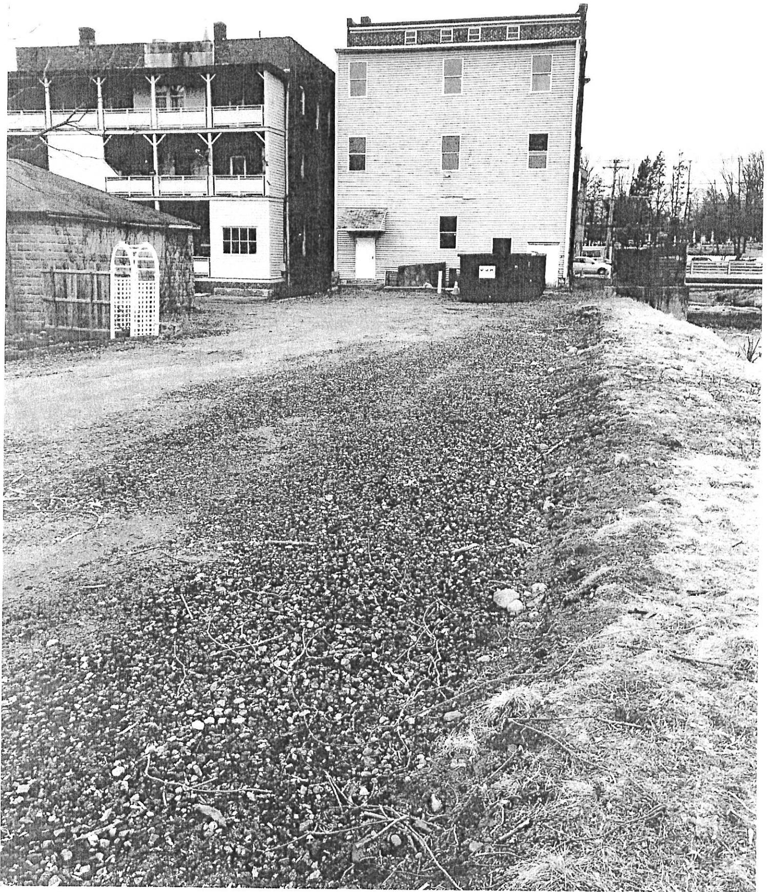
2-18-20 120 East Main St
