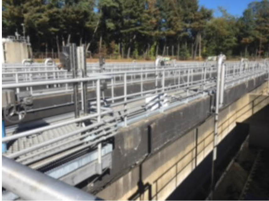
Sample #3 @ Aeration Tank Number 1
