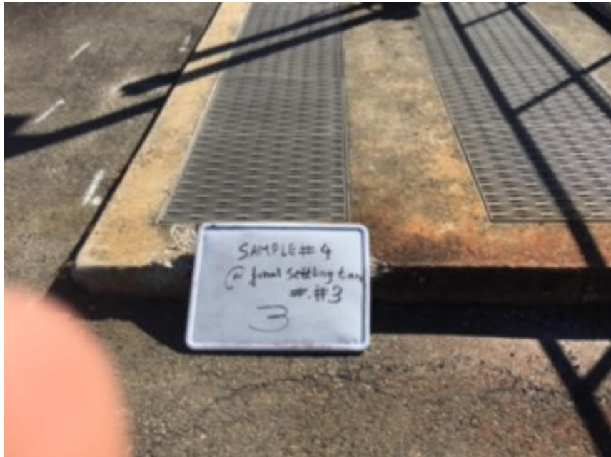
Sample #4 @ Final Settling Tank Number 3
