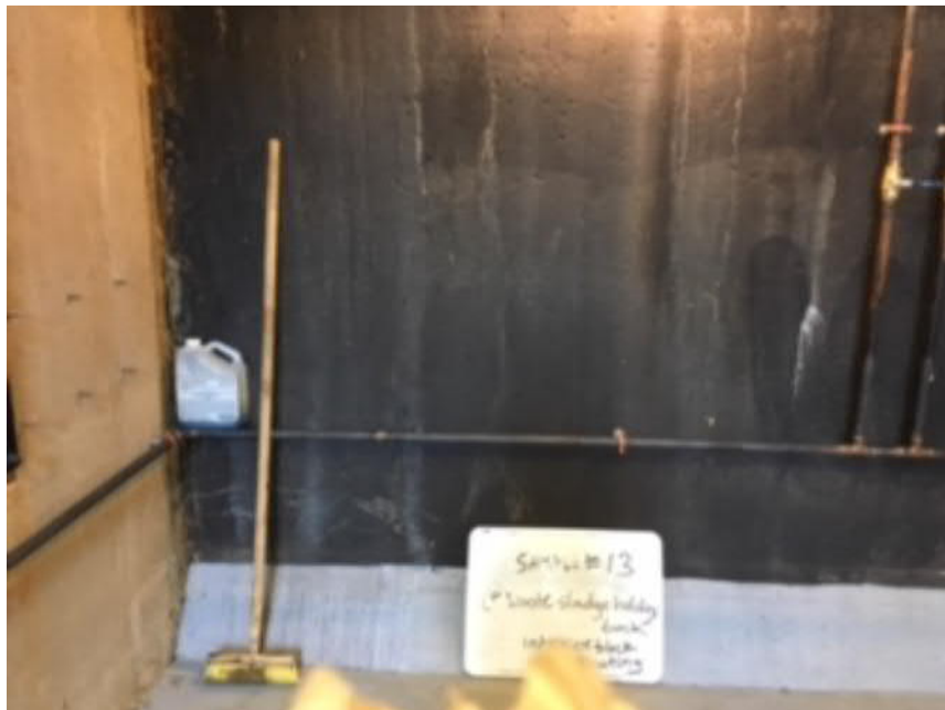
Sample #13 @ Waste Sludge Holding Tank (Exterior wall - Interior access)
