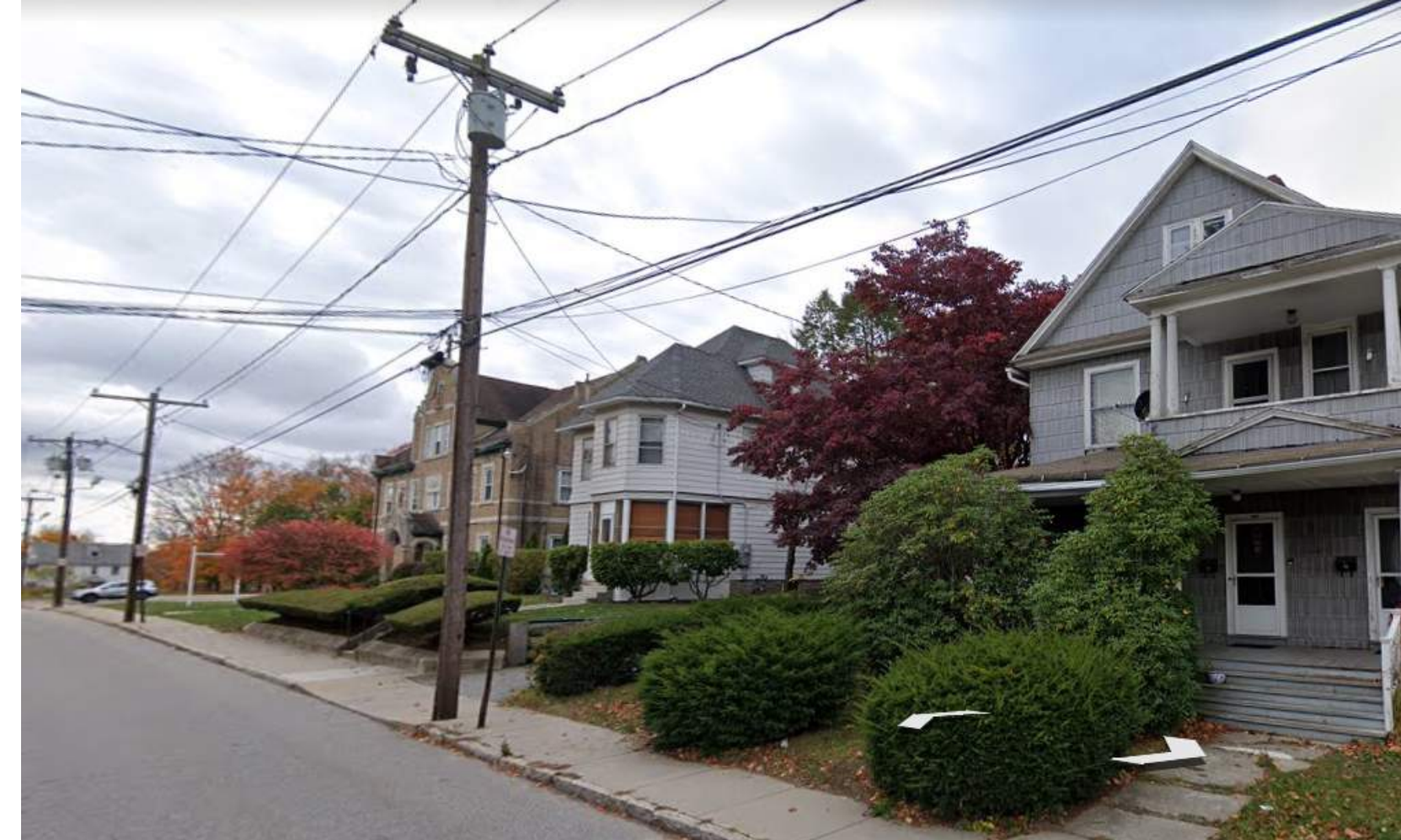
GROVE STREET CONVENT ADJACENT BUILDING - NORTH SIDE
