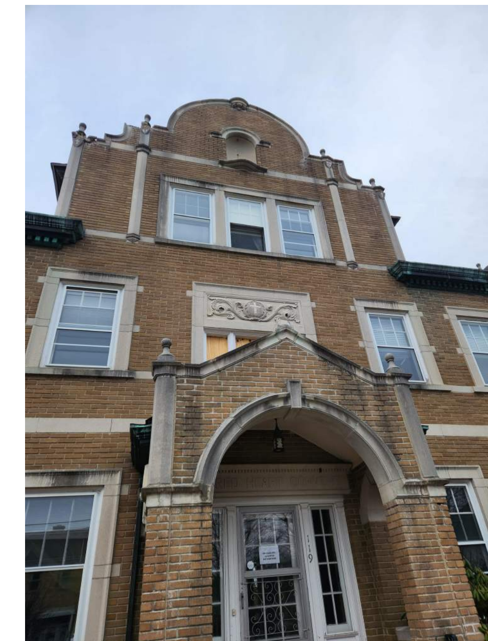
CONVENT MAIN BUILDING WEST ELEVATION
