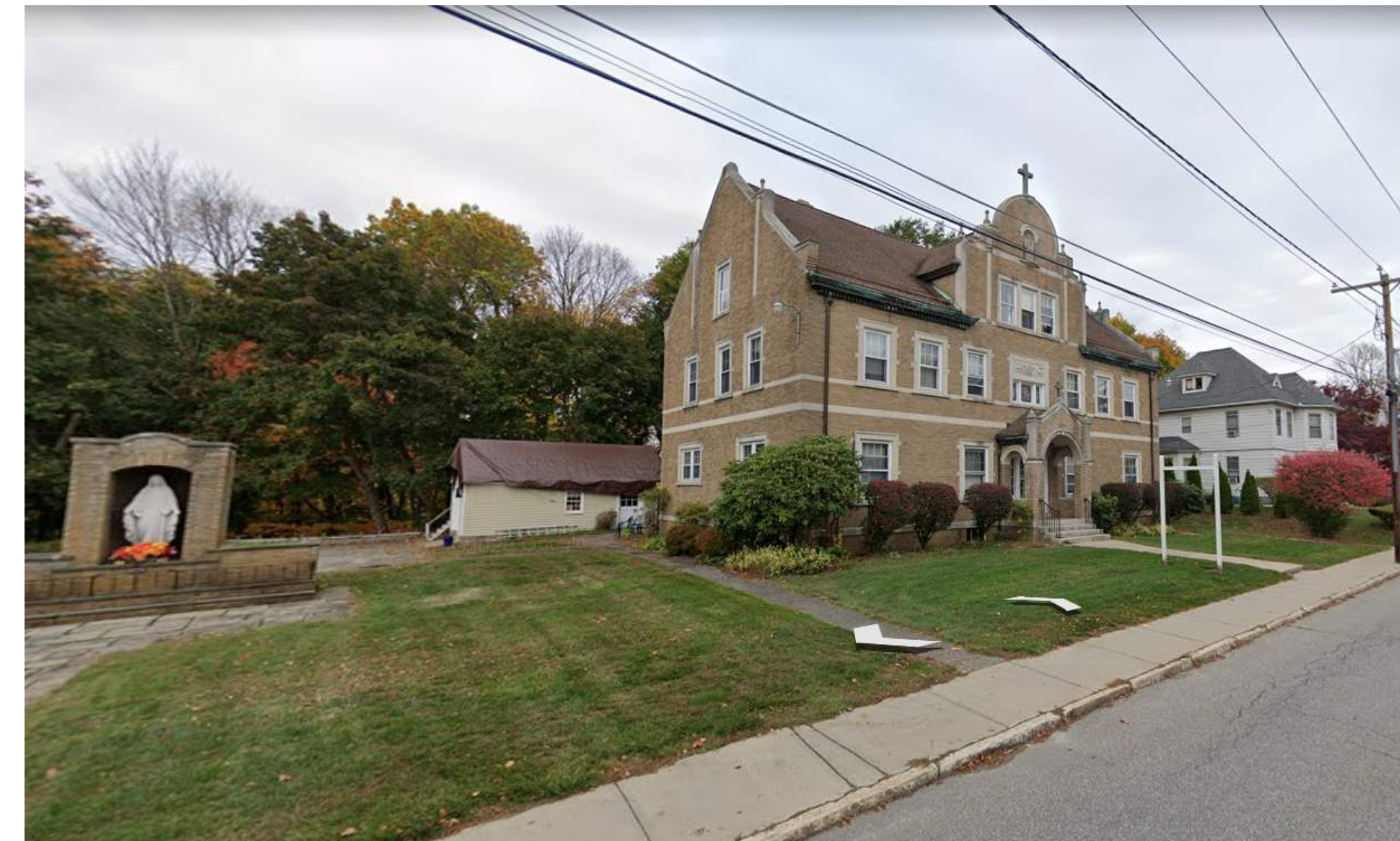
GROVE STREET VIEW CONVENT MAIN BUILDING LOOKING SOUTH WEST
