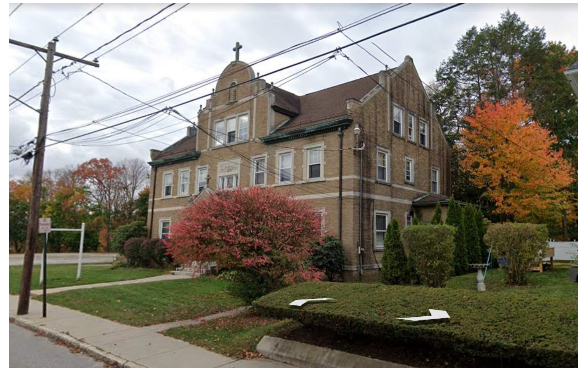
GROVE STREET VIEW CONVENT MAIN BUILDING LOOKING NORTH WEST
