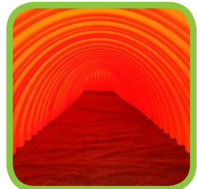
Looking down the Isolator Row from the manhole opening, woven geotextile is shown between the chamber and stone base.
