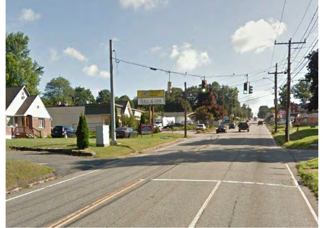
Safe Pedestrian Facilities Lacking Throughout Corridor
