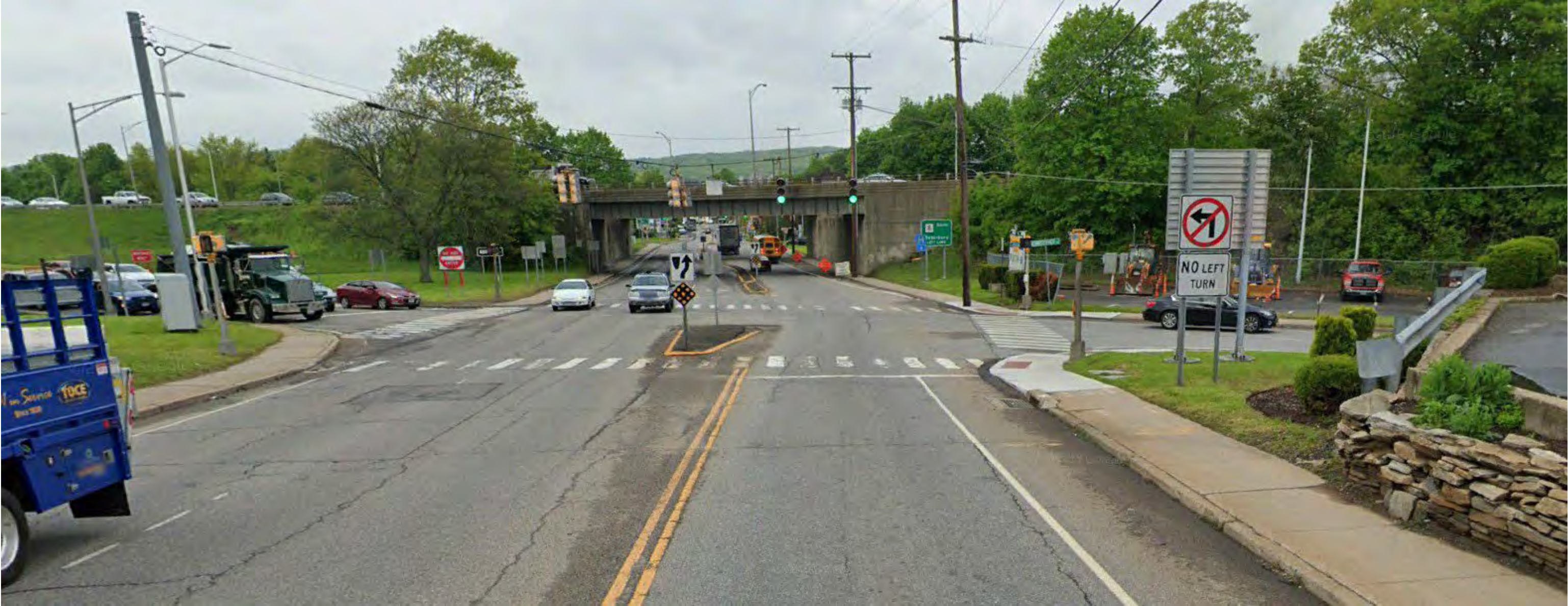
Existing View at Route 8 Gateway
