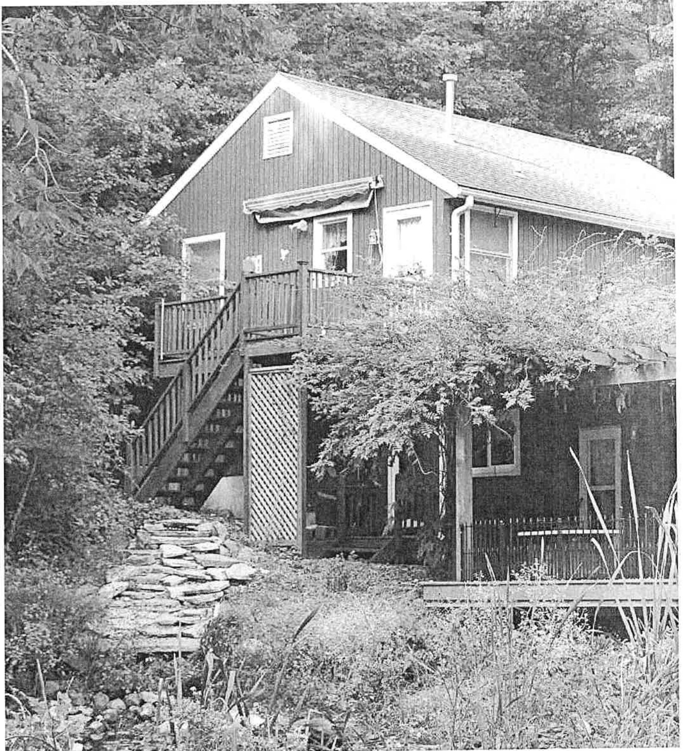
A Connecticut home with an accessory apartment as seen in 2016. File photo
