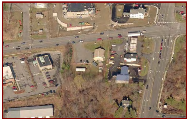
Intersection of Route 189 and Route 200
