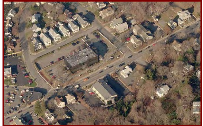
The Glass Building on Route 208/4
