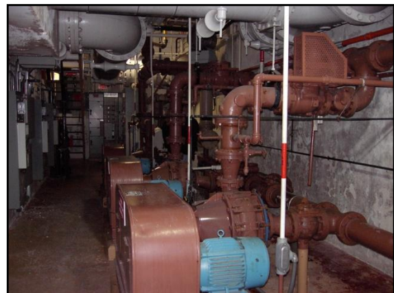
Recessed Impeller Grit Pumps
