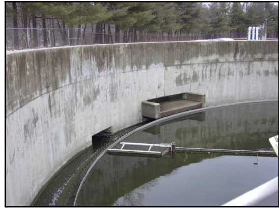
Final Settling Tank Overflow Structure
