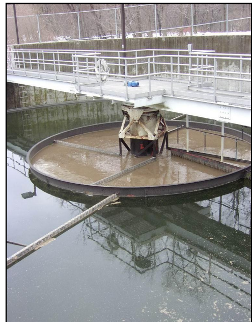
Circular Final Settling Tank
