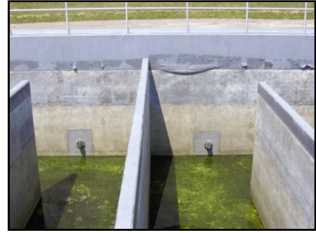
Chlorine Contact Tank Coating Failure
