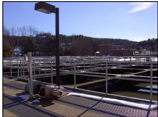
Primary Settling Tanks
