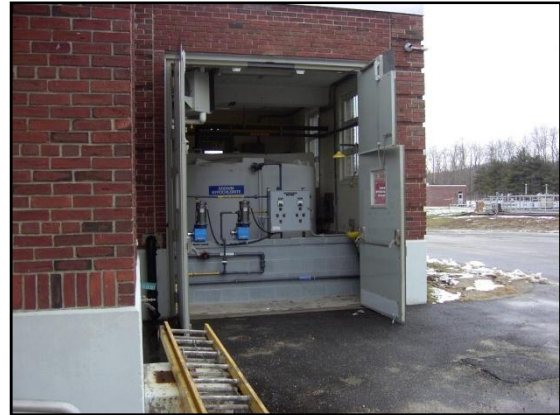
Sodium Hypochlorite System
